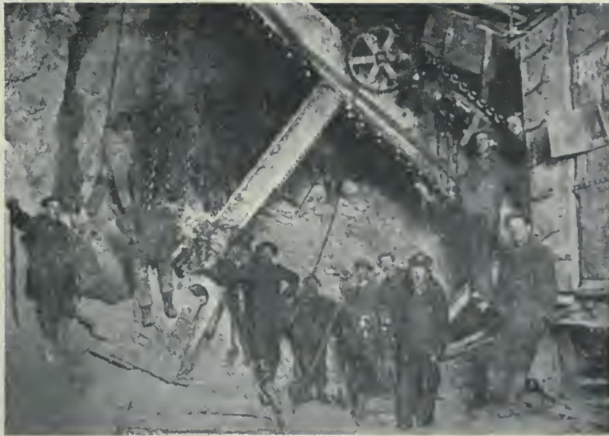
Steam Shovel averages 50 ft. a day in enlarging Rogers Pass Tunnel
